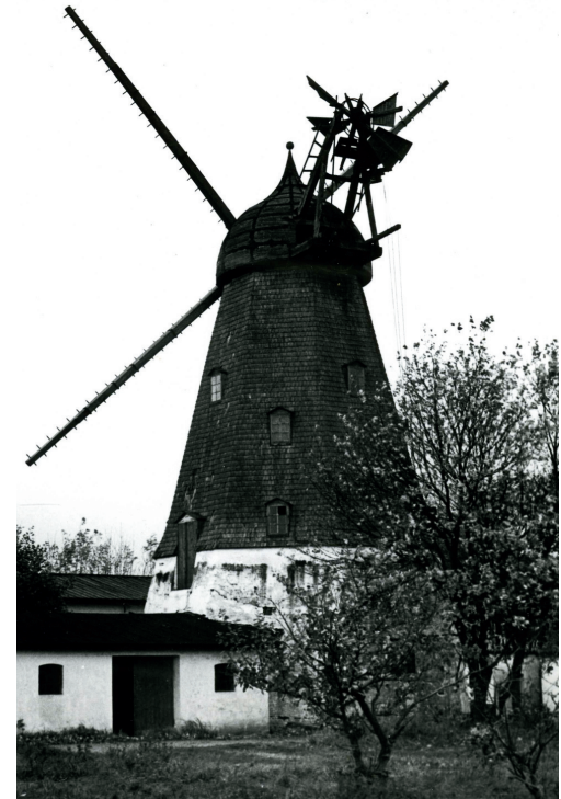
The windmill in disrepair, 1975
